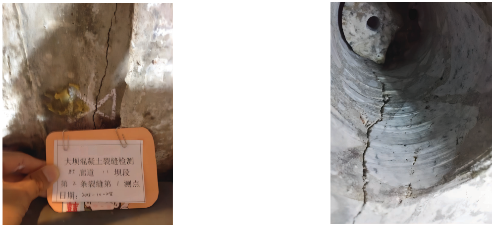
Figure 1. Field detection photos of typical cracks.
