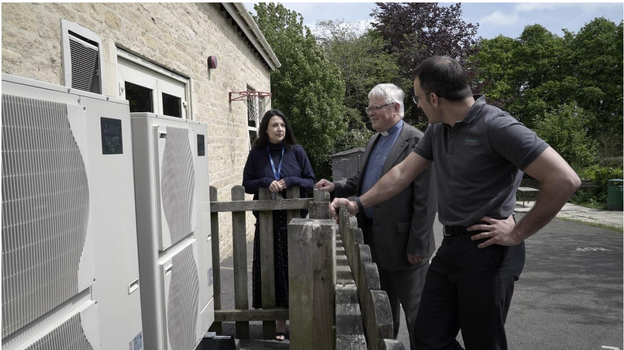
Heat Pumps at St Andrew's Primary School, Chedworth, now a net zero carbon school
