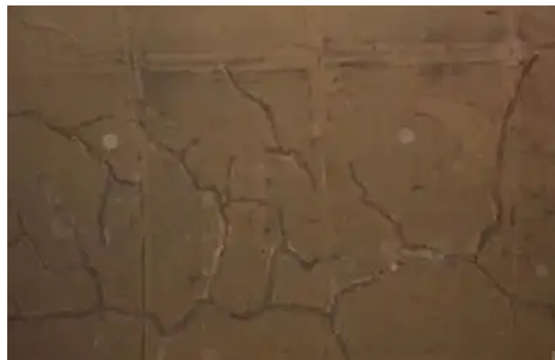
Figure 1. Reticulated cracks in the secondary lining
