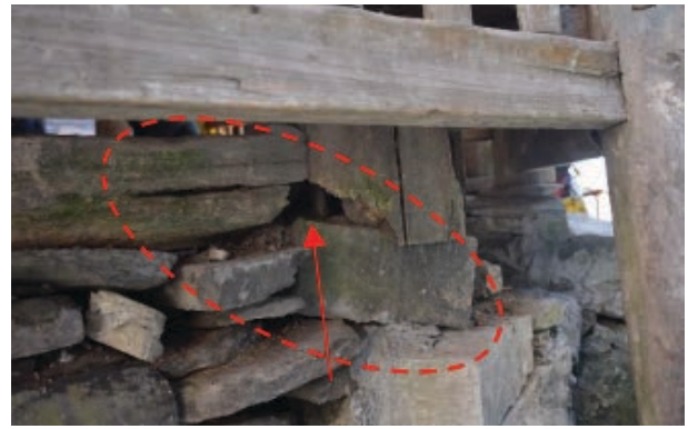
(b) Biological degradation at column bases
